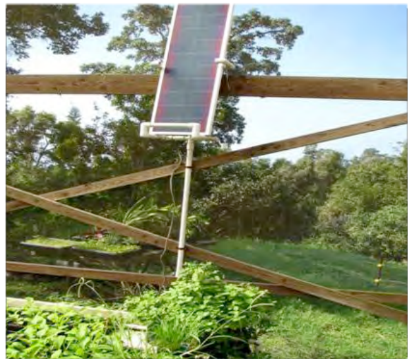
Solar panel driving irrigation table pump. Pump slows or turns off when cloudy and plant water demand is lower.
