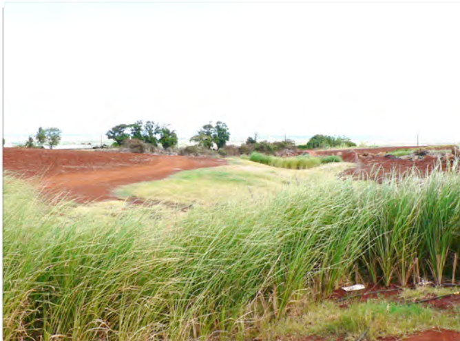
'Sunshine' vetiver grass is used with Bermudagrass to stabilize a waterway in Kunia.
