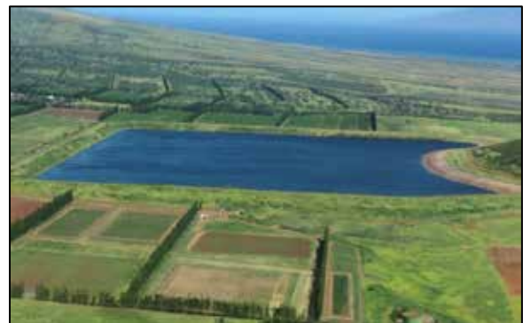
Molokai Irrigation System, presently managed by the State Department of Agriculture, is the lifeblood of the Molokai farming community.
