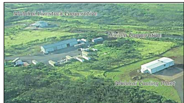
Agricultural infrastructure in the Molokai Agriculture Park. Two of these facilities, Molokai Livestock Cooperative and Molokai Cooling Cooperative were constructed as part of the Extension Community Resource and Economic Development Program.
