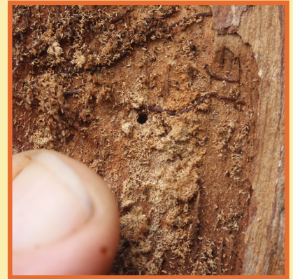
Fine beetle boring dust around a boring hole.
