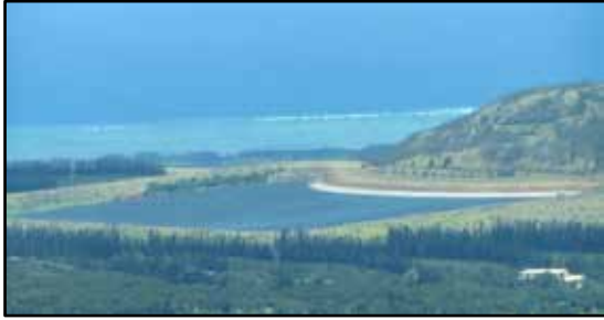
The 124-acre Molokai Irrigation System Reservoir in Kualapu'u
