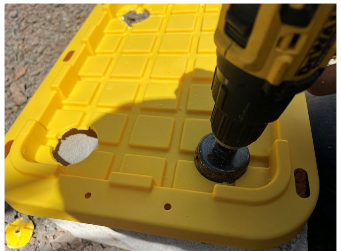
Photo 3. A two-inch hole saw was used to drill holes for the net pot.
