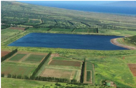
Molokai Irrigation System, life blood of the farming effort in Ho'olehua, Molokai. Managed by the State Department of Agriculture, this 124-acre reservoir holds 1.4 billion gallons at full capacity. Water originates from Waikolu Valley on the north shore of Molokai.
