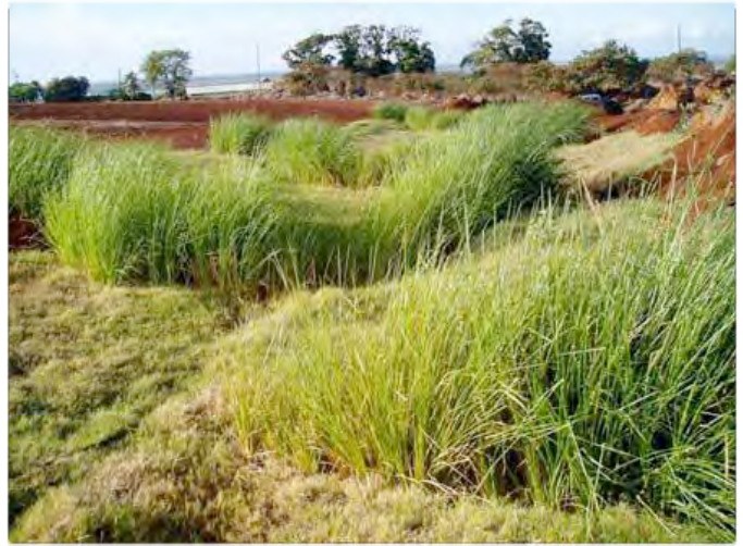
Vetiver is used in combination with Bermuda grass to stabilize a drainage path.
