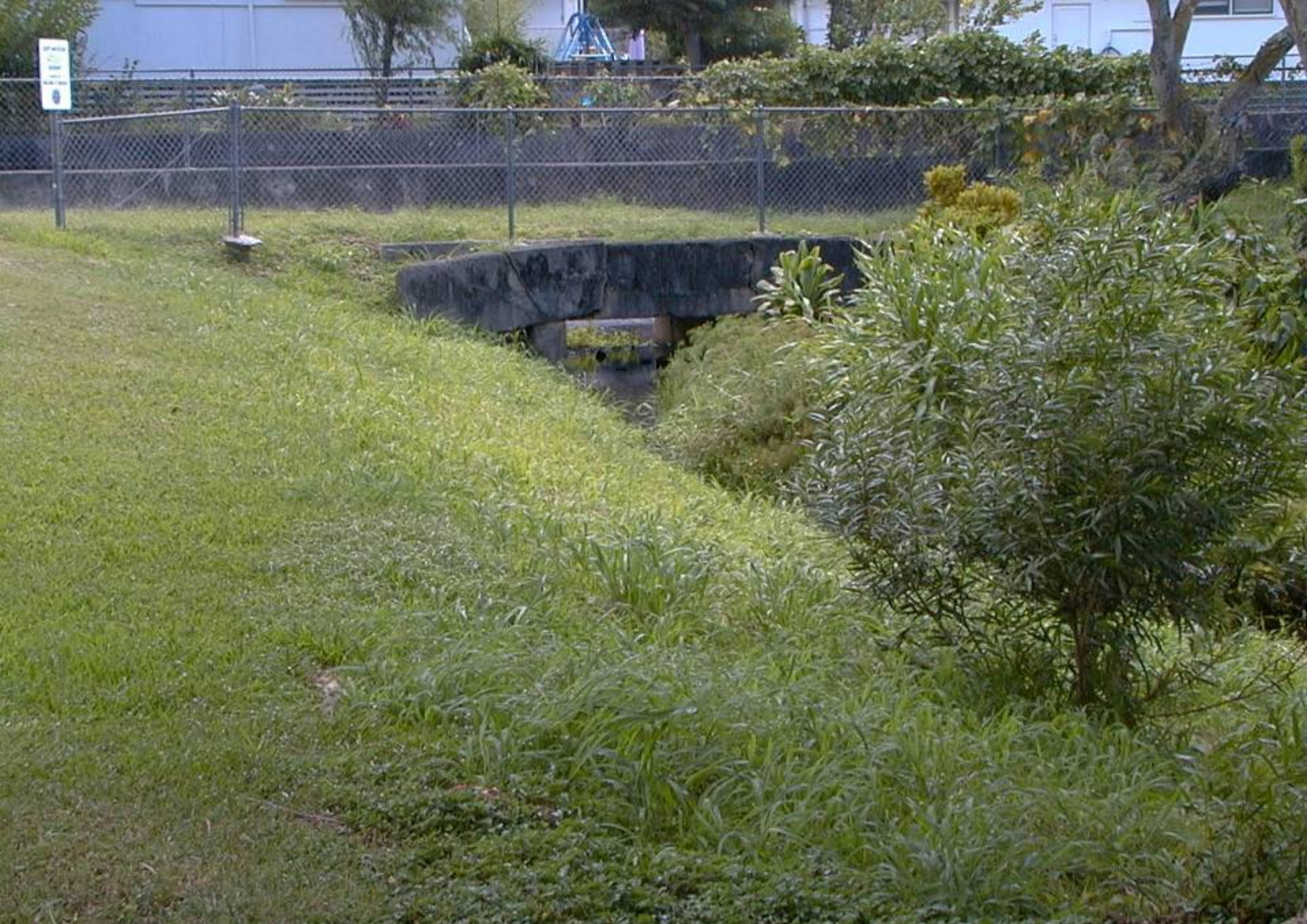
Drainage near Manoa Elementary School
