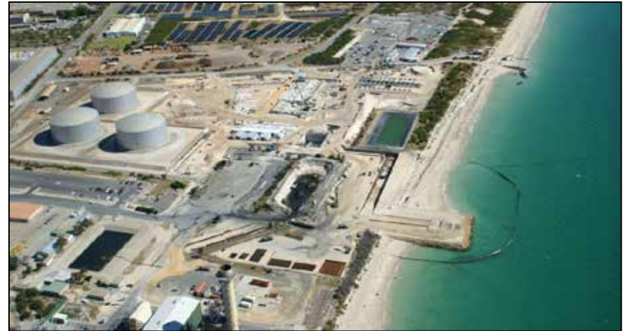
Perth Desal. Plant will be largest in S. Hemisphere
