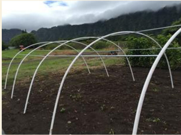
EMT conduits to support PVC pipes.
