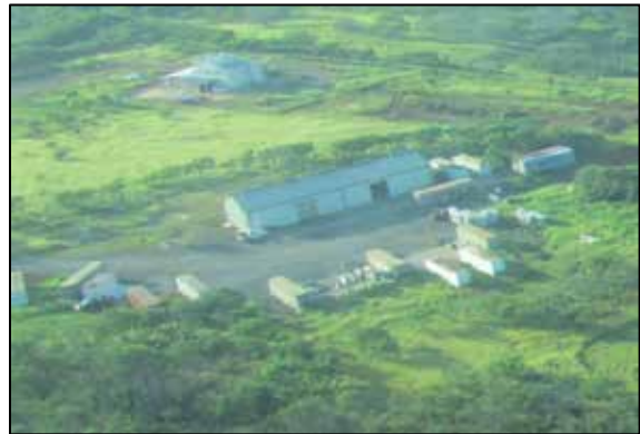
Molokai Livestock Cooperative slaughter facility (background) and Hikiola Cooperative, a farm supply cooperative founded by Hoolehua Hawaiian Homesteaders in 1976. We've worked closely in the development and/or expansion of these cooperatives.
