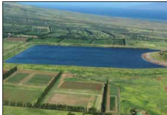
An engineering feat, the Molokai Irrigation System transports water from Waikolu Valley on North Molokai through a 5 mile tunnel to this 124 acre reservoir in Kualapuu that can hold 1.4 billion gallons of water on a good day.
