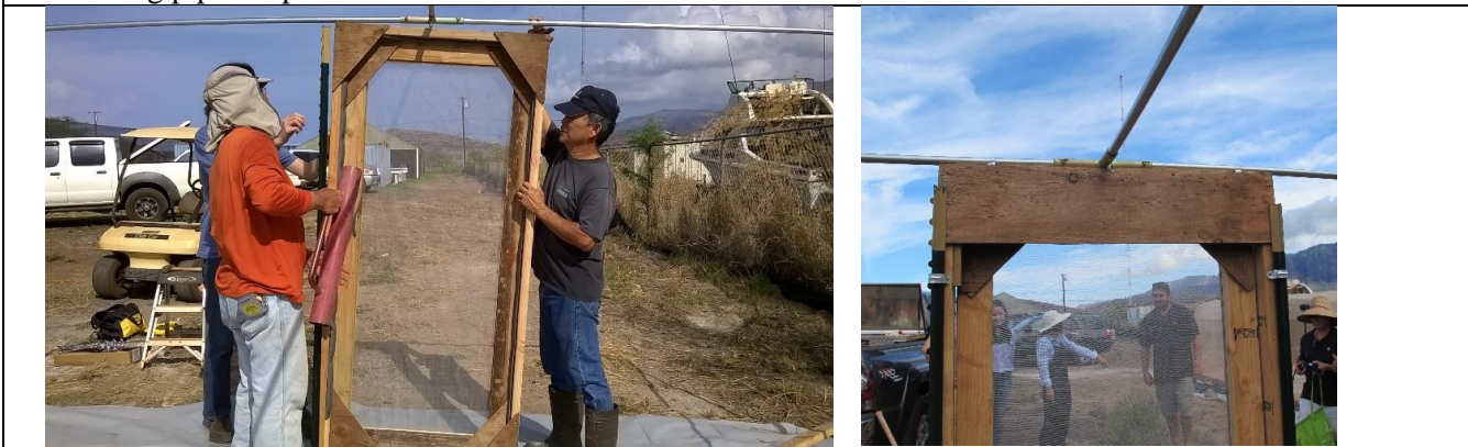
Erect a door anchored with 2 T-posts pounded into the ground and secured to the door jamb with pipe straps.
