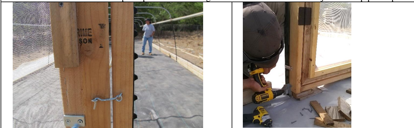
Door is installed and attached to T-posts using 1" pipe straps. Secure door to the rest of the frame with
