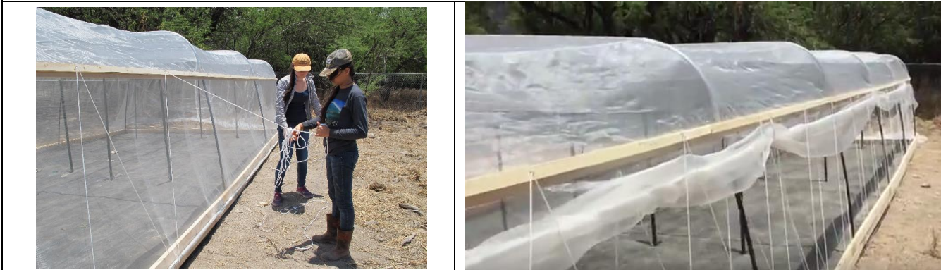
Thread one billow twine through the eye screws outside and one inside of the retractable screen.
