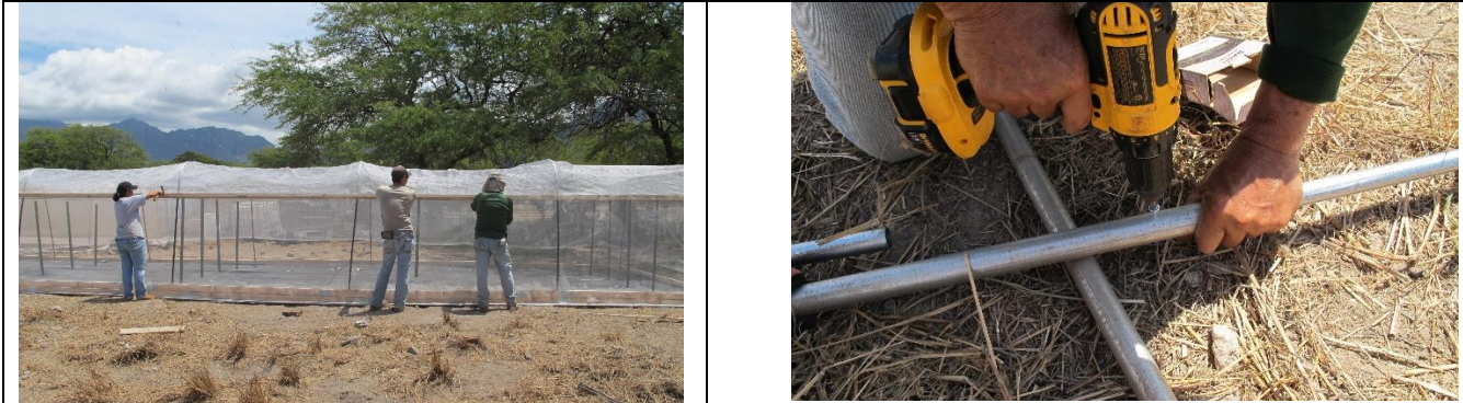
Securing the frame for the top of the retractable wall.
